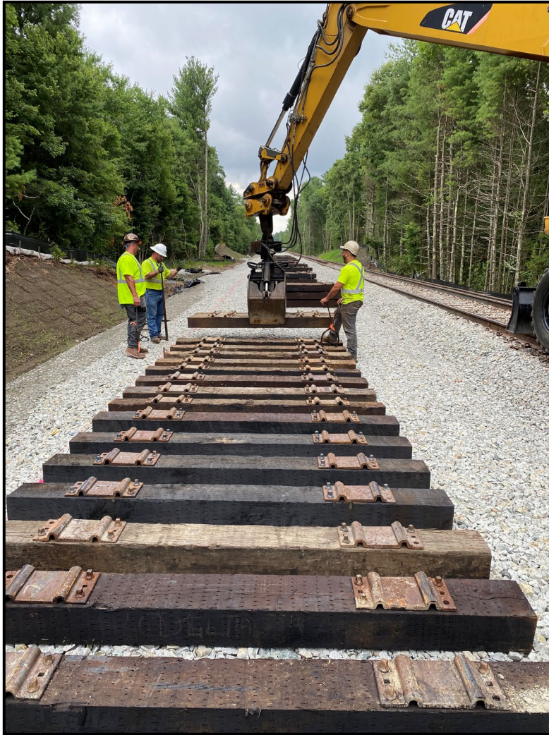
Laying ties near Padelford Street in Berkley, August 2022
