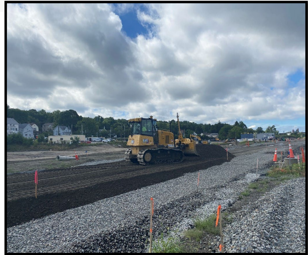
Weaver's Cove Layover prep for paved access to rail yard, August 2022
