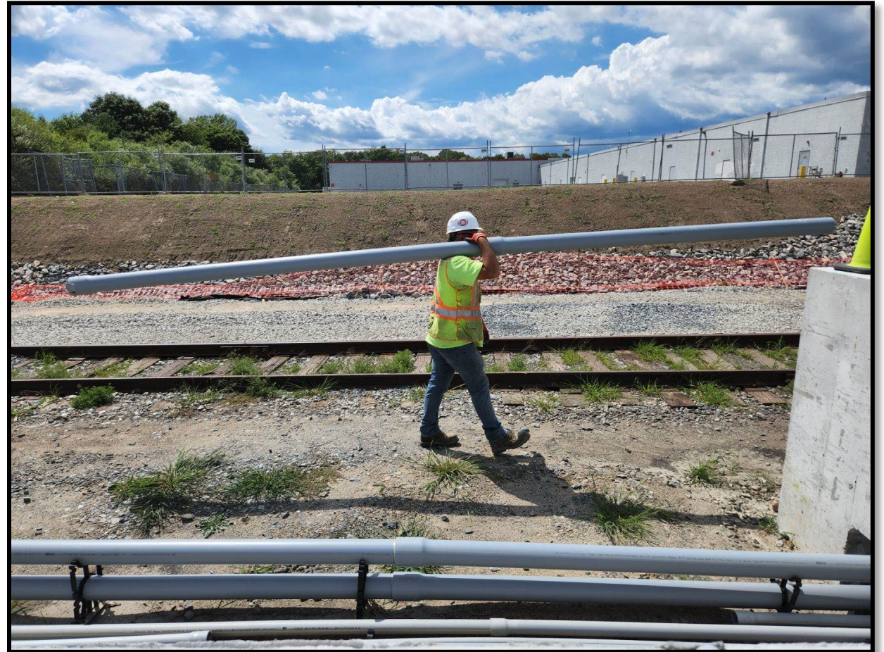
Installing conduits under platform at Church Street Station, August 2022
