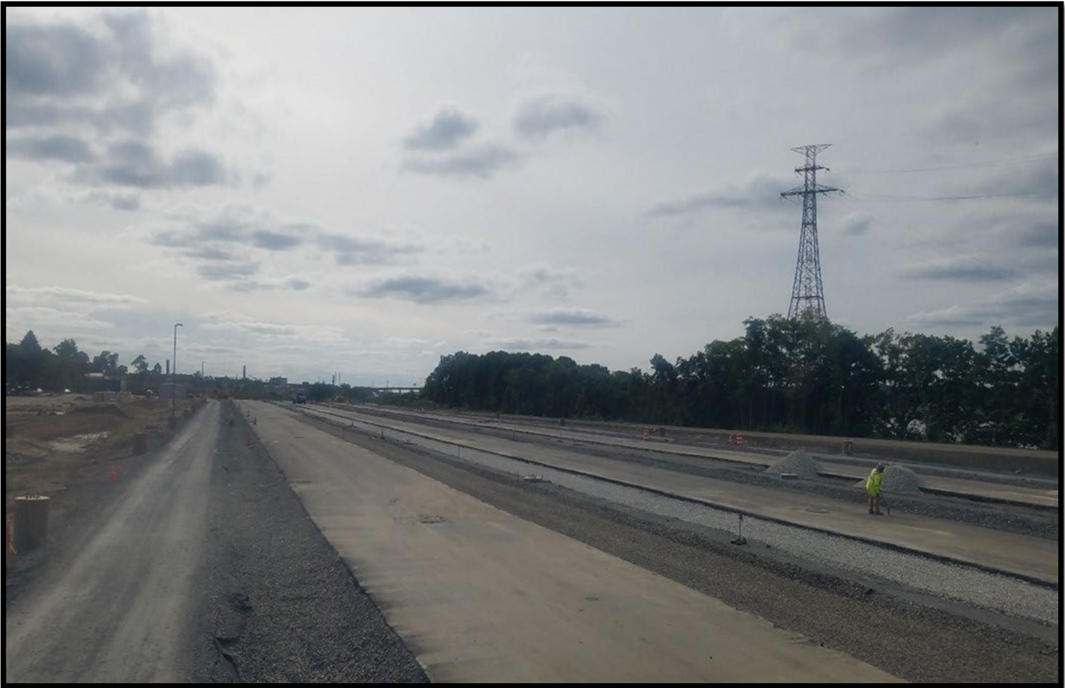
View south of yard area, September 2022
