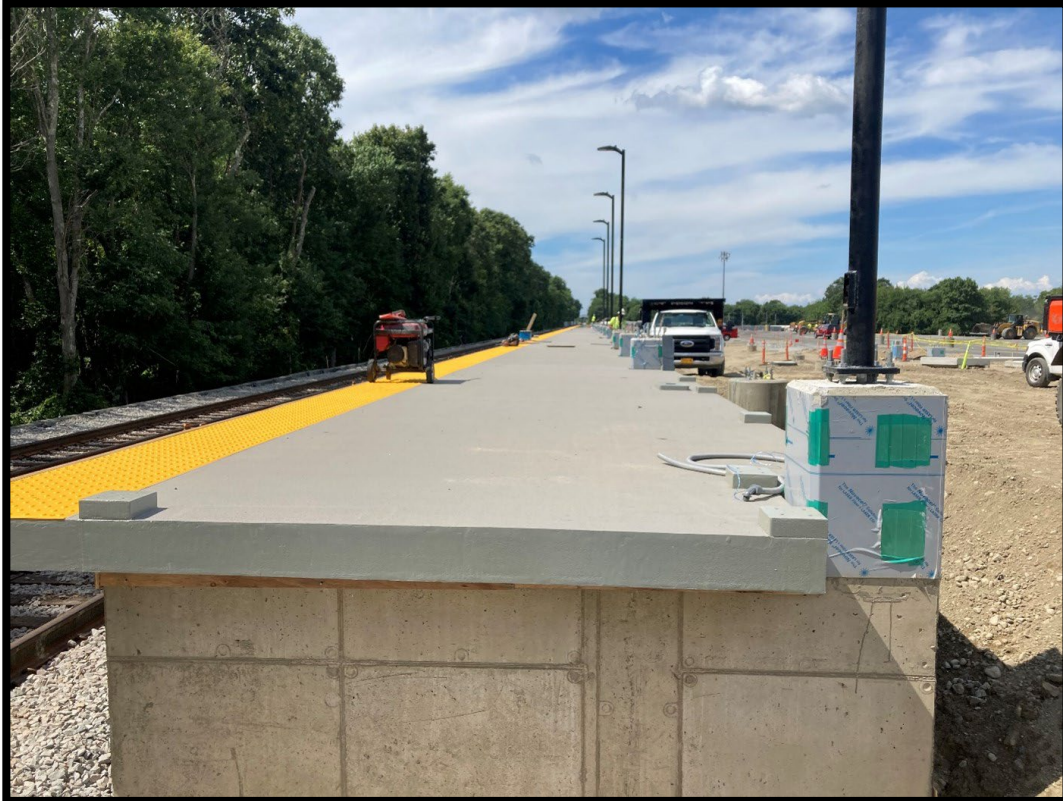
Freetown Station platform light pole installations, August 2022
