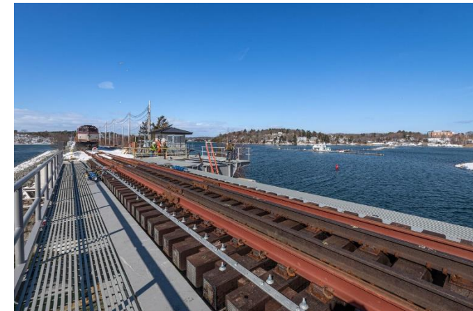
New ties and track on the Gloucester Drawbridge
