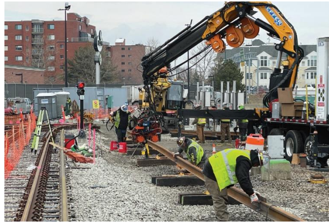
Installing new track in Wellington Yard
