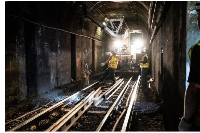
Track, signal, and power upgrades on the Blue Line
