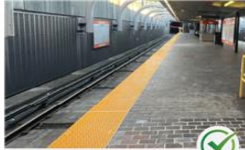
Ruggles Station Tactile Replacement
