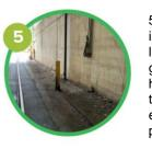
5. Clogged **weep holes** in retaining walls can lead to increased groundwater and higher hydrostatic pressure on the wall. This may be exacerbated by extreme precipitation.
