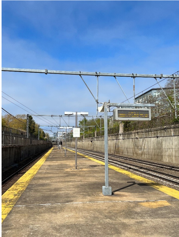
Existing platform requires accessibility upgrades
