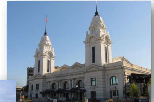
Worcester Union Station
