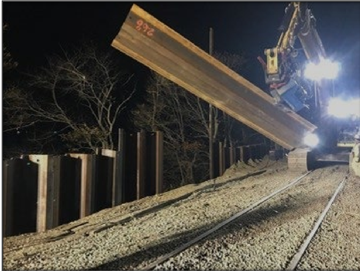
Installation of sheet piles
