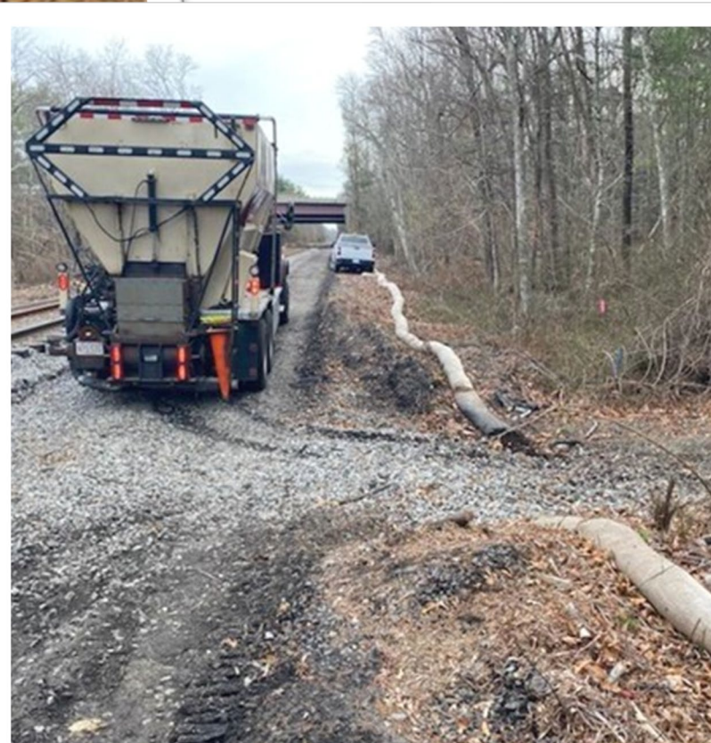
Erosion controls along the ROW
