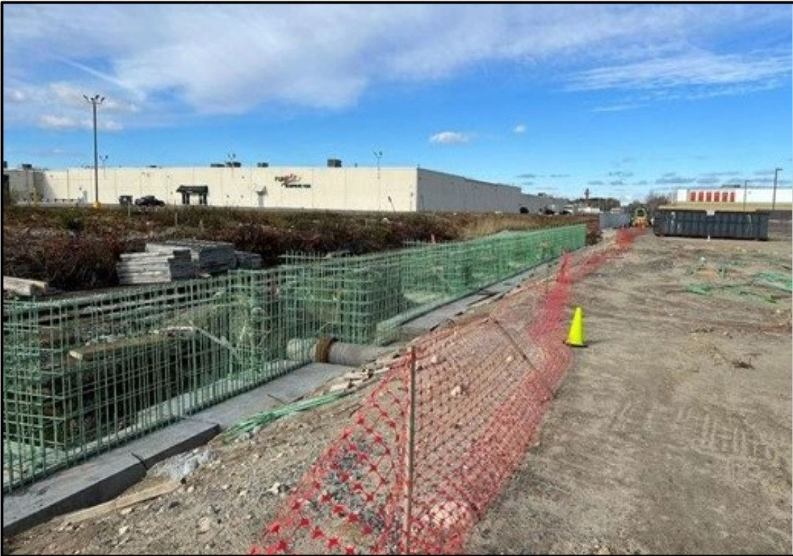
Church Street platform walls formwork and reinforcing steel, December 2021
