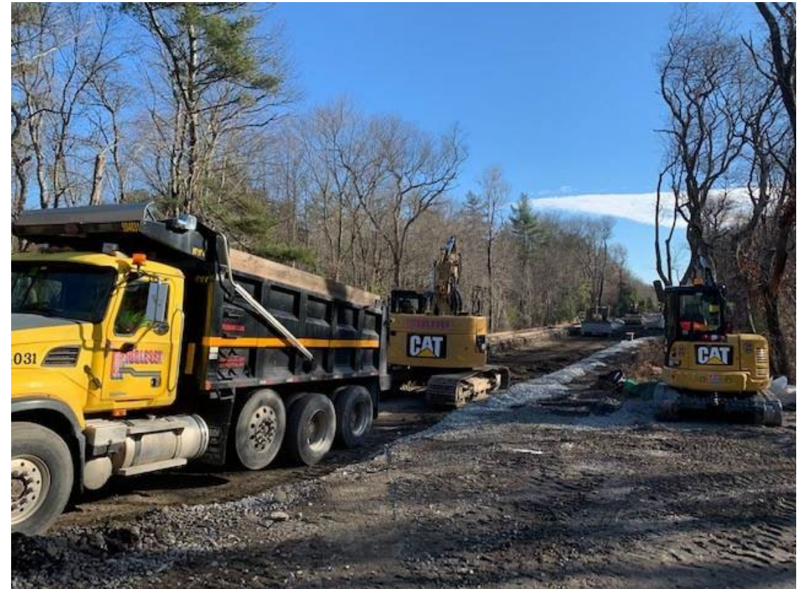
ROW work, New Bedford Jan 2022
