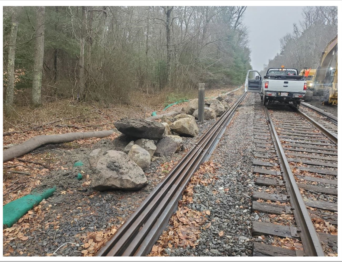
Right of Way work, New Bedford, January 2022
