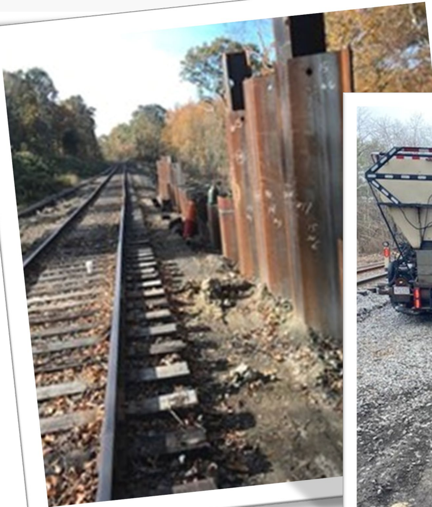
Ongoing sheet pile detail work
