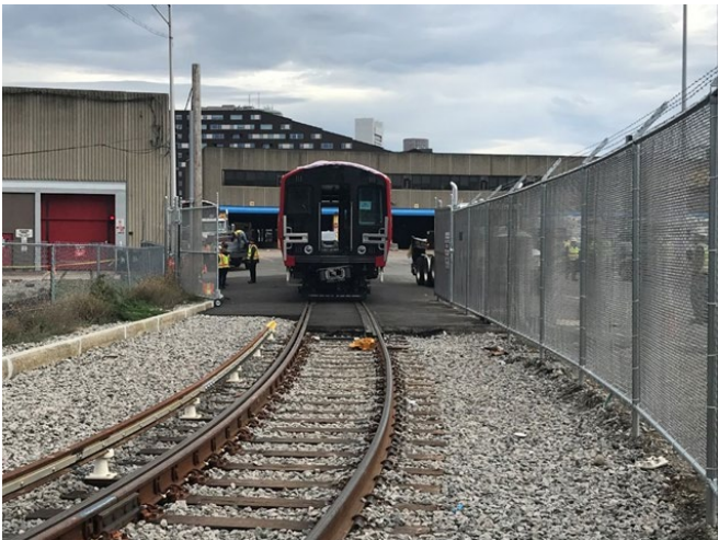
Completed construction of a new 4,500 (TF) Test Track for new Red Line Vehicle delivery and testing.
