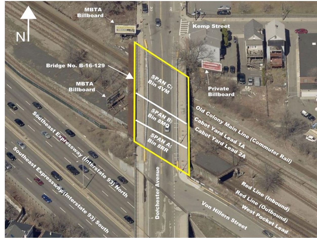
Close up view of the Dorchester Ave. Bridge
