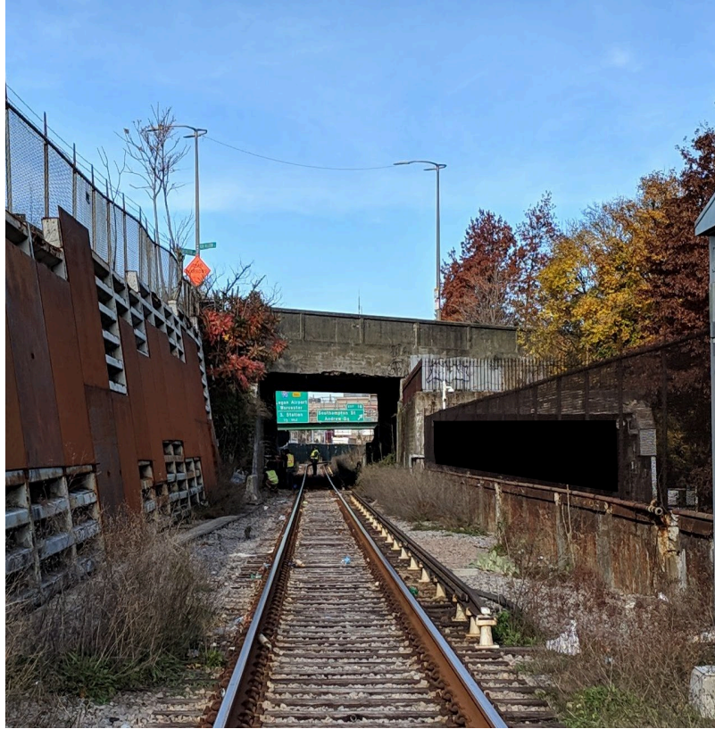
Red Line Track - East Elevation Von Hillern Street Retaining Wall on the left
