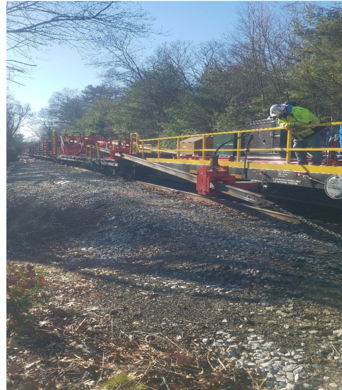
Offloading 1600-foot rails
