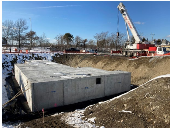
Fall River Depot stormwater detention tank
