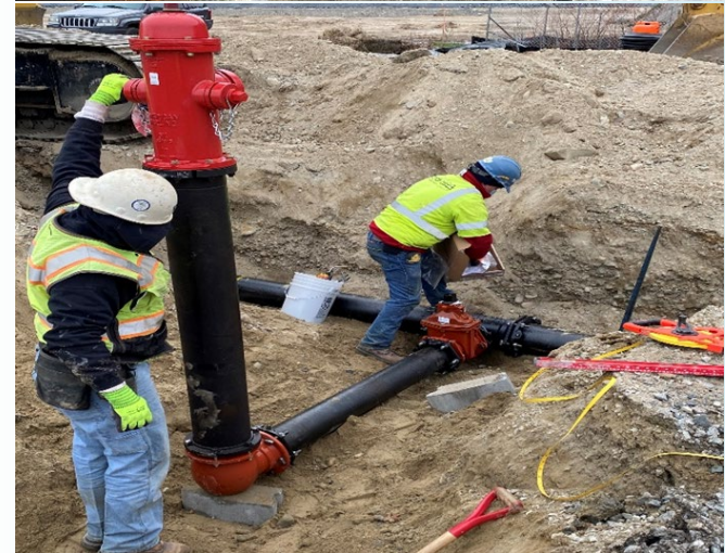
Hydrant installation at Weaver's Cove
