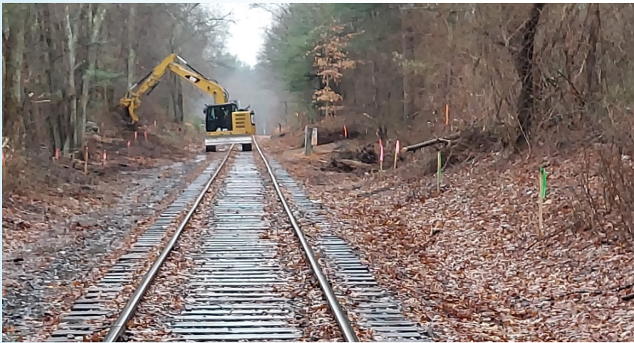
Top – clearing and grubbing along the right-of-way
