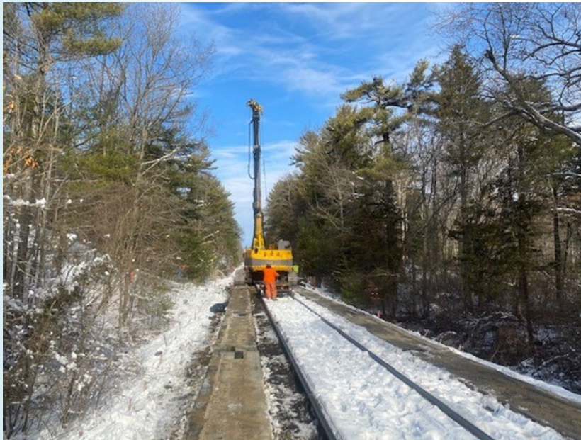
Installing sheet piles (above); installing platform micropiles for the station (right)
