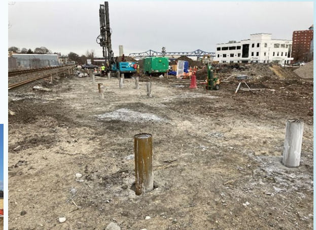
Fall River Depot – micropiles installed for station support
