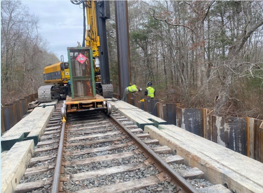
Marine sheet piles being installed (above) and in place (top right)
