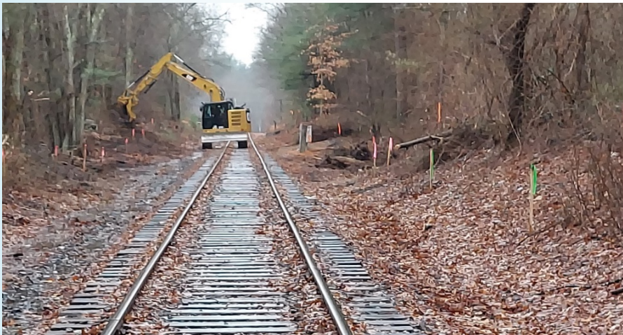
Clearing and grubbing along the right-of-way
