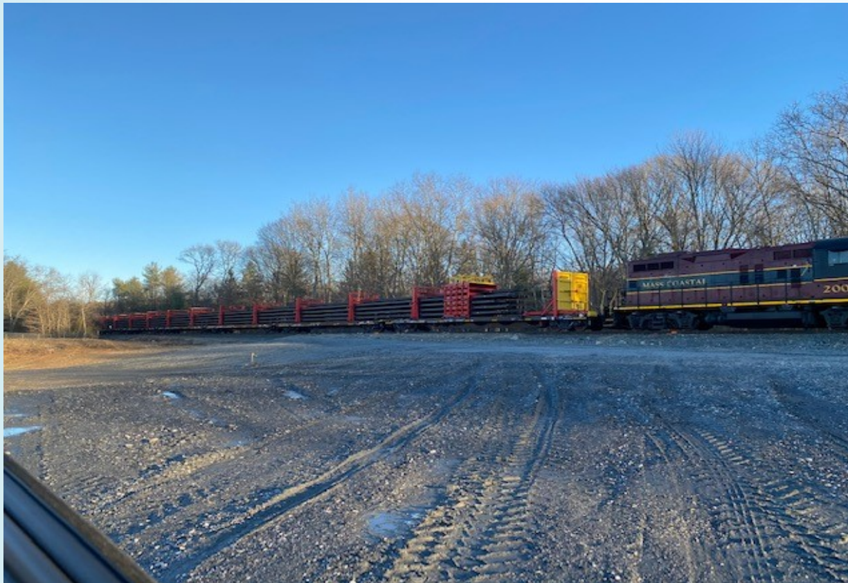
Offloading 1600-foot lengths of rail (Freetown)
