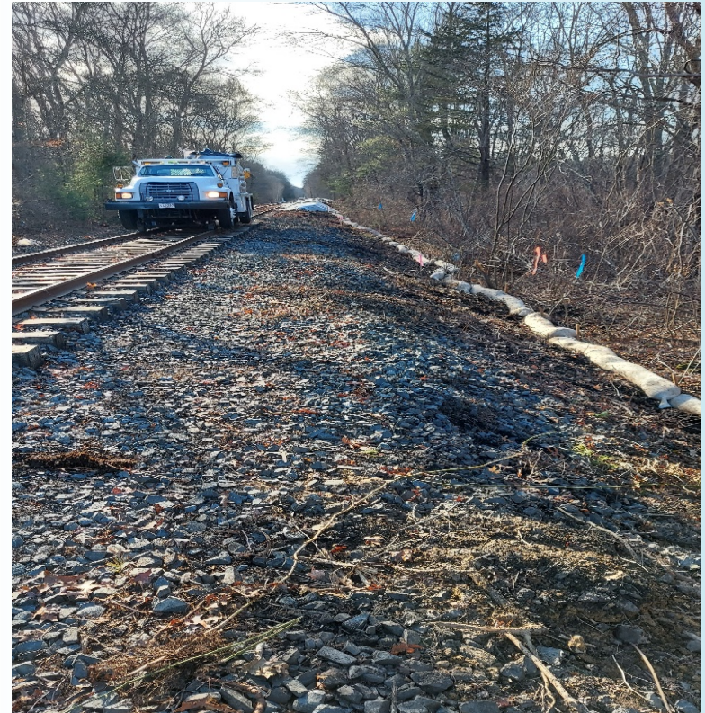
Installing erosion protection (example)
