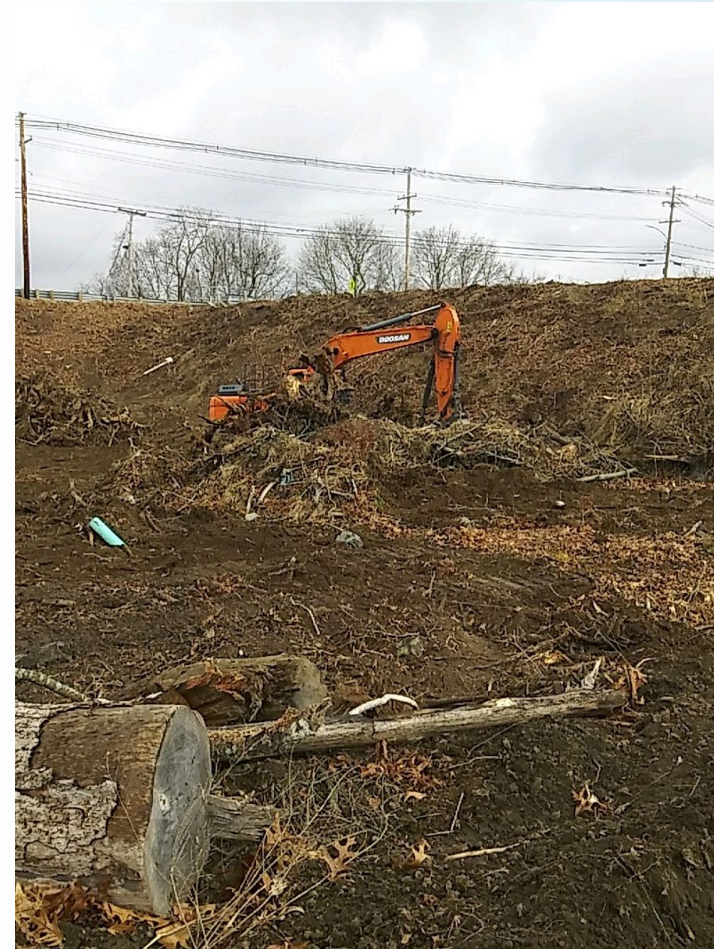
Site clearing, Middleborough Station
