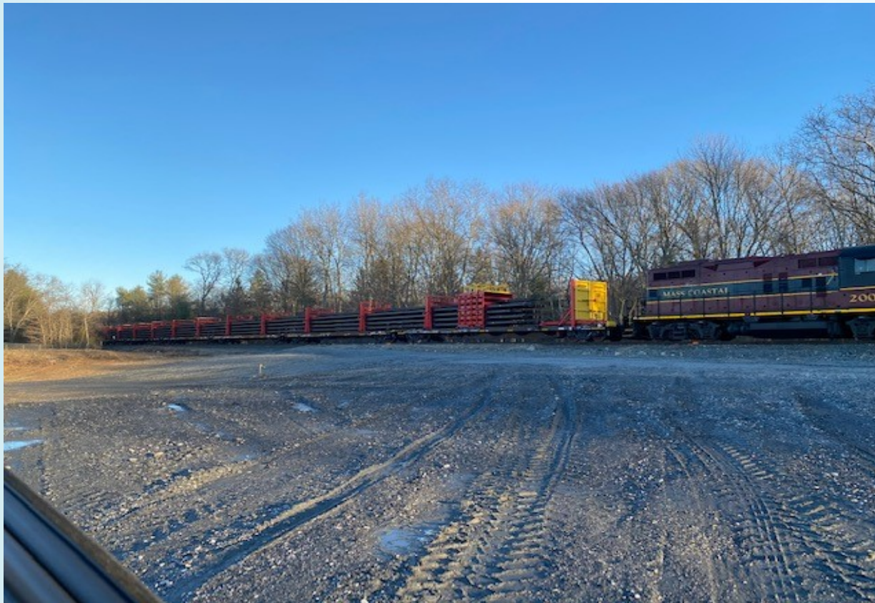
Offloading 1600-foot lengths of rail (Freetown)
