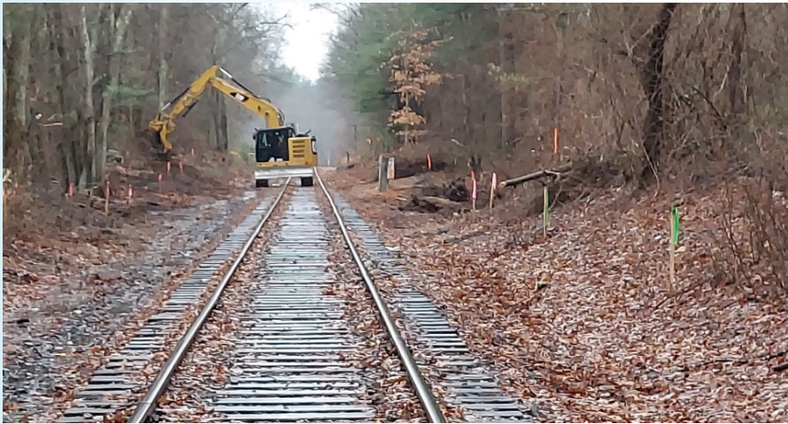
Top – clearing and grubbing along the right-of-way
