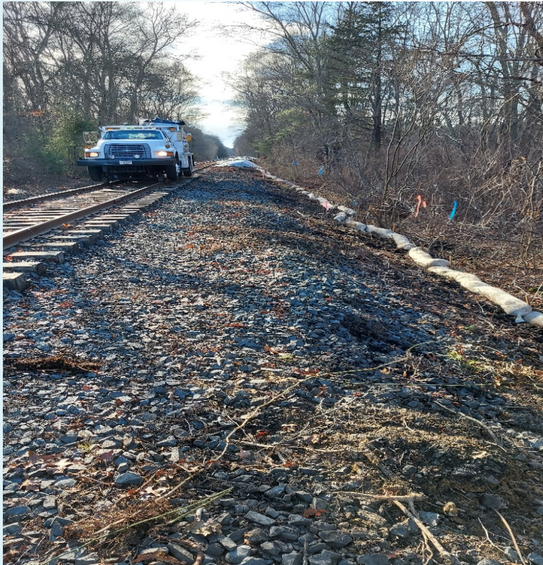
Installing erosion protection (example)
