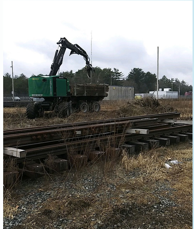
Right - Site clearing at Middleborough Station
