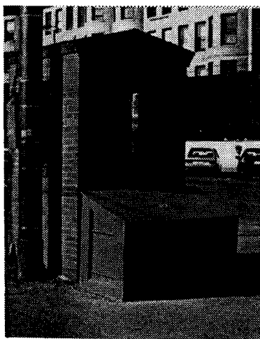
Fig. 2-108 Existing Sand Storage Bin
