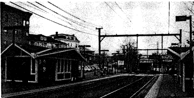
Fig. 2-120 Existing Wood Shelter at Brookline Village
