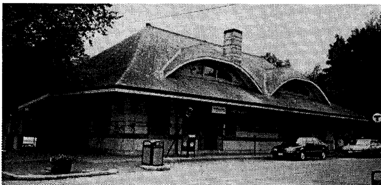
Fig. 2-117 Existing Shelter at Newton Center Station
