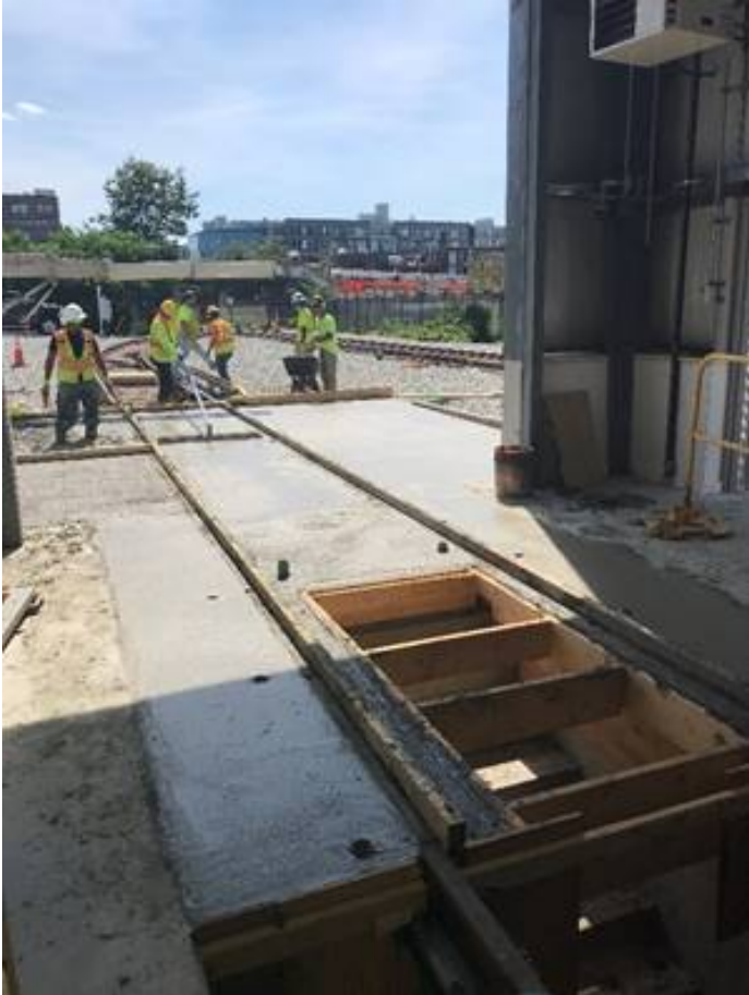
Red Line Test Track: VTF Concrete Placement at South Apron
