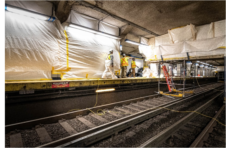
Blue Line: State Street Asbestos Removal
