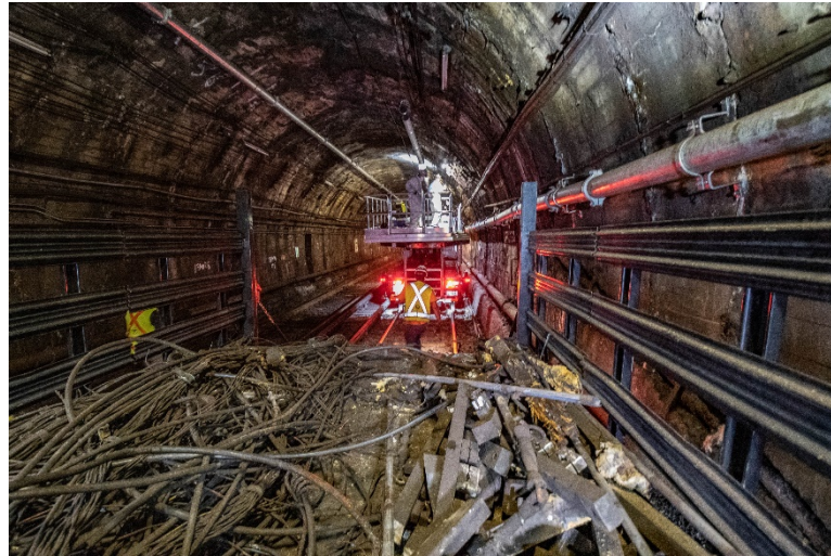
Blue Line Cable Removal
