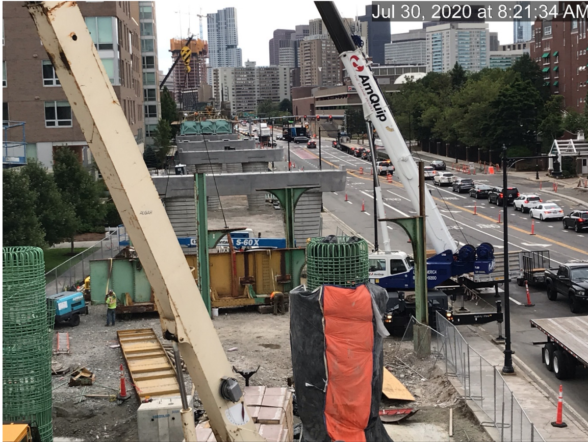
Steel being removed from old Lechmere viaduct structure.
