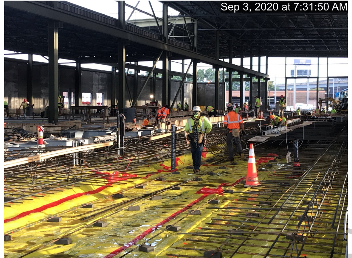
Reinforcing steel in VMF floor.
