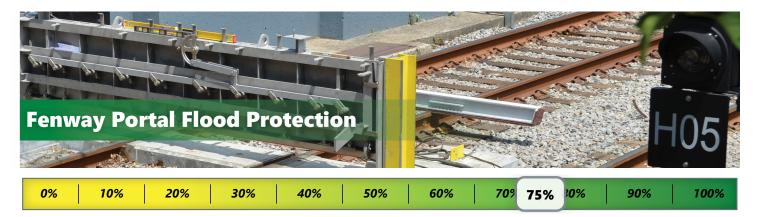
Addition of large steel doors to the Fenway tunnel entrance to prevent future flooding
