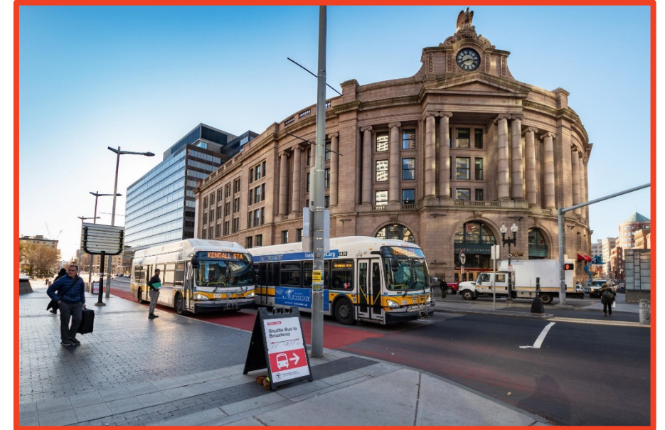
Photo of Red Line Diversion
