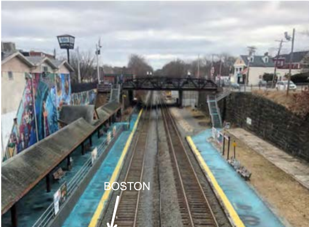
Photo of Existing Conditions
