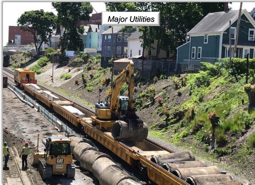
Sub surface drainage work continues (existing and new)
