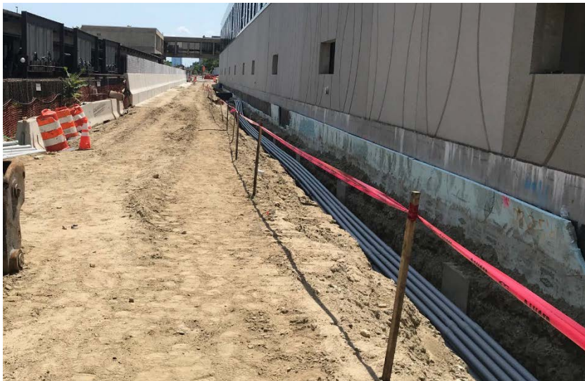
New fence installed on barrier (L) and duct bank (R) at East Access Road
