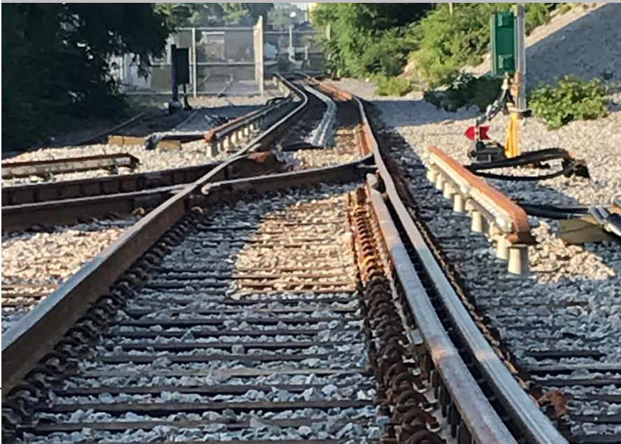
Installed Third Rail Insulators Leading into Turnout
