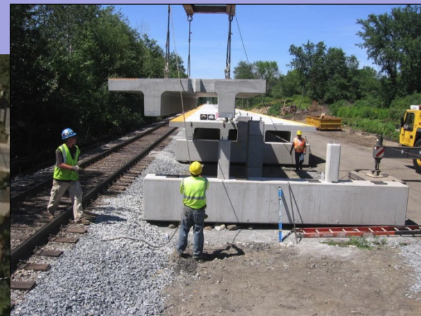
Precast Elements Assembled
