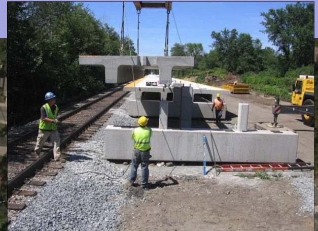
Precast Elements Assembled
