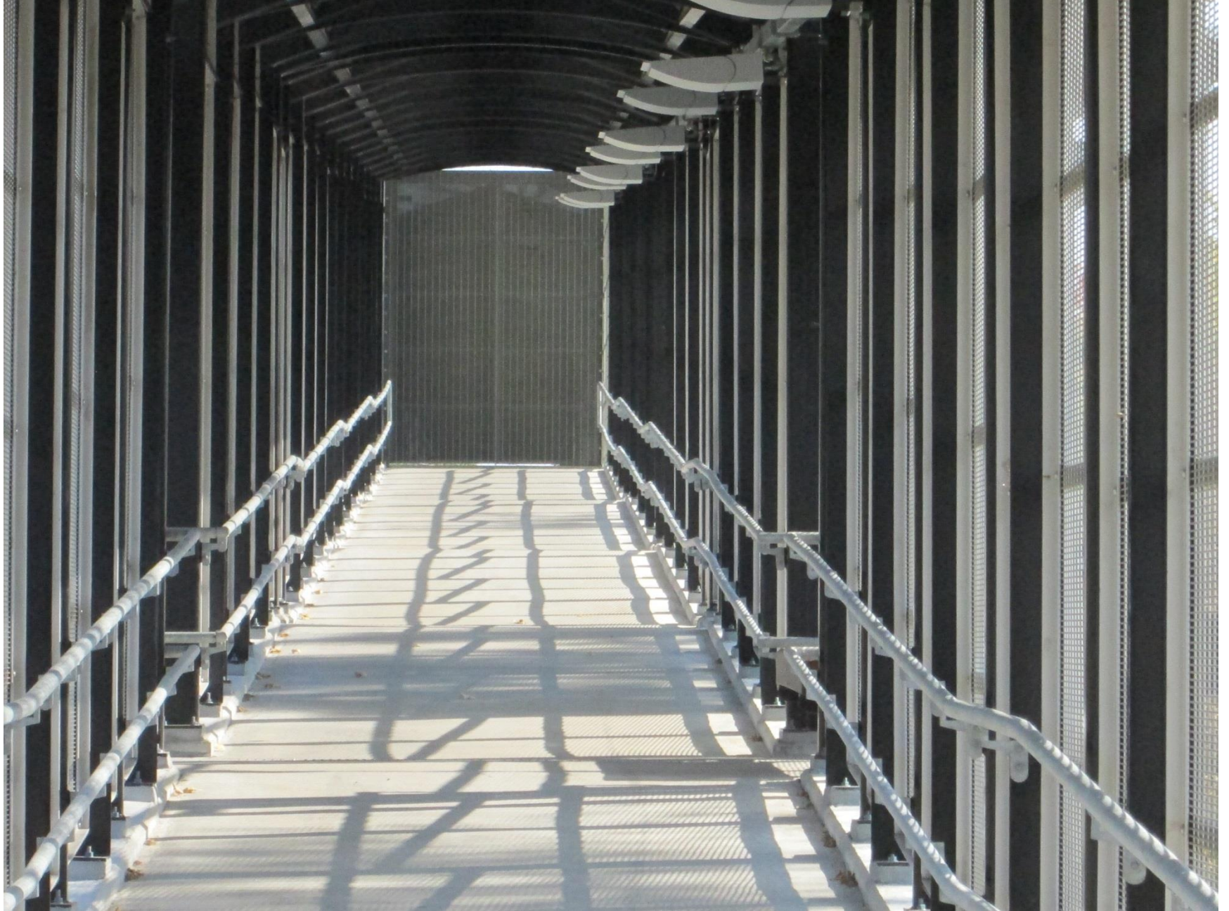
LITTLETON STATION (Typical view inside ramp structure)
