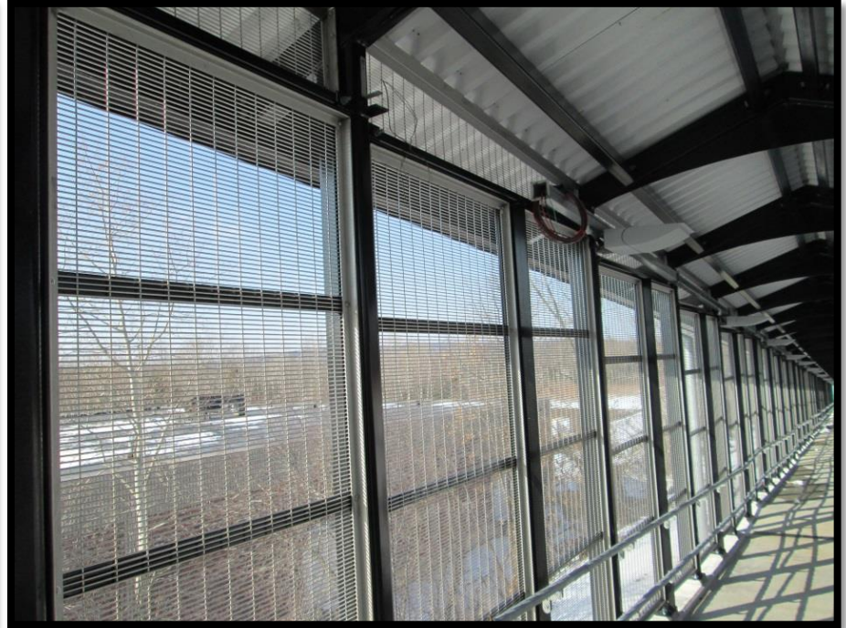
LITTLETON STATION (view out ramp structure)
