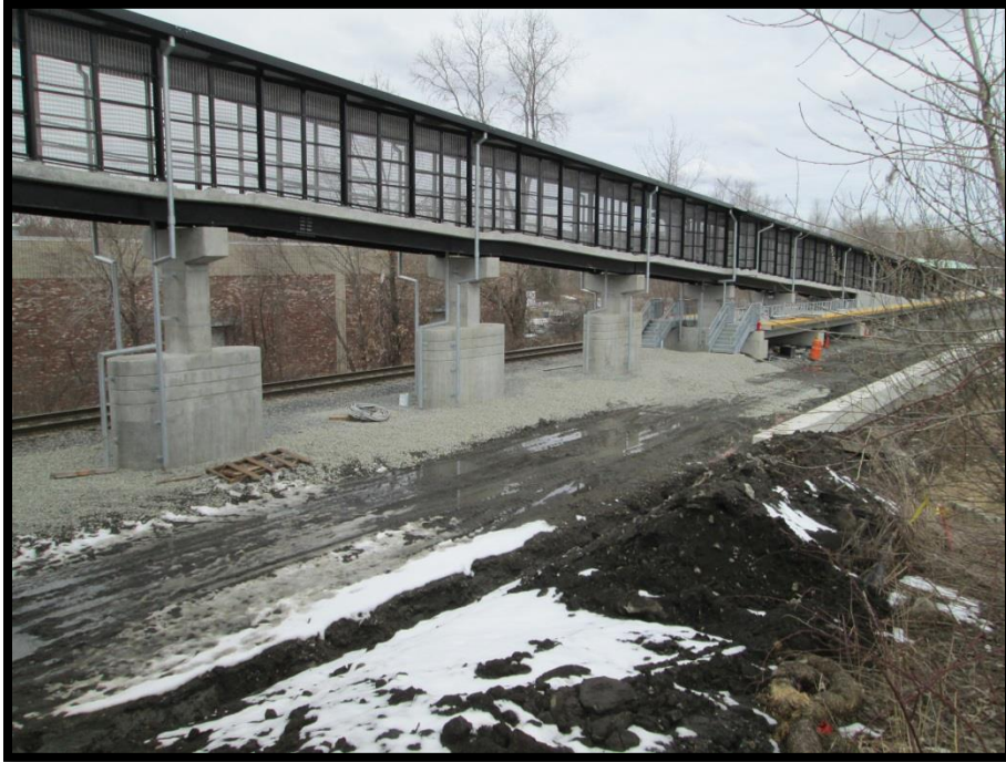
LITTLETON STATION (view towards ramp)
